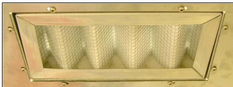
2. Remove the filter by gripping the filter itself, and pulling straight down. (As shown below.)
